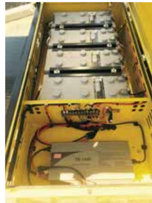
Main Panel: Battery, Power Inverter & Switch
